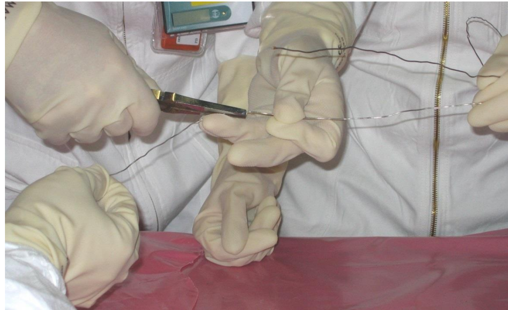
Repairing a mineral insulated cable
