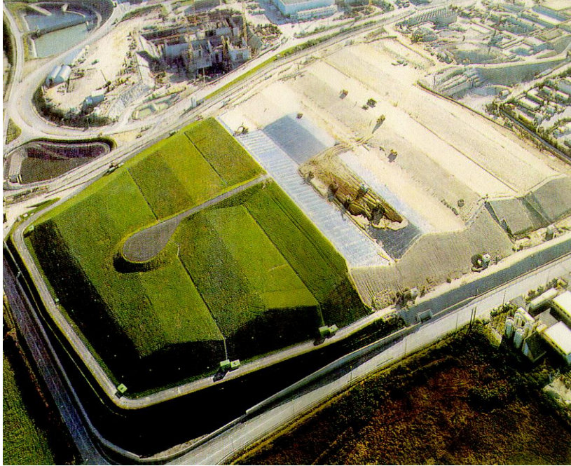
Final covering of LLW disposal facility Centre de la Manche, France
