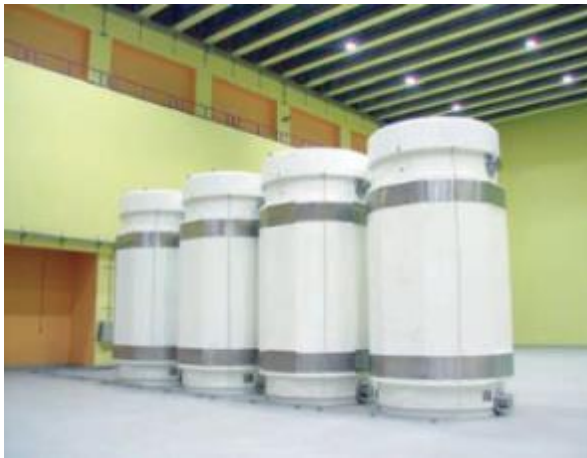
Dry storage casks
