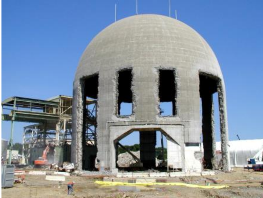
Maine Yankee being dismantled, USA
