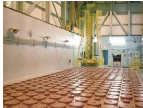
Dry storage building
