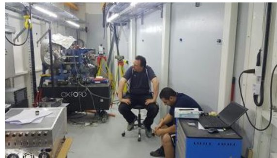
Alignment of the DCM & Other components
