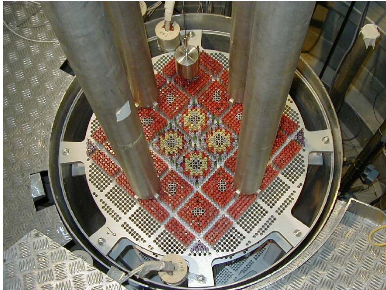
Top view of the EOLE reactor core
