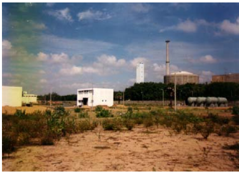
Fig. 5. Hybrid (MSF+RO) plant, Kalpakkam, India
