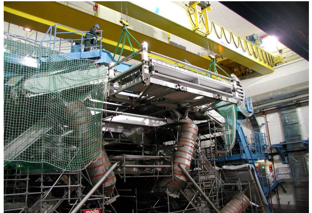
Installation of barrel muon station (40% done)
