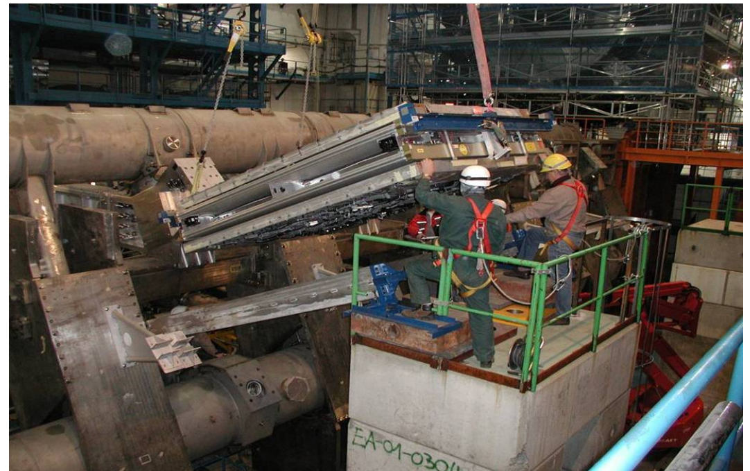
Installation of barrel muon station (40% done)
