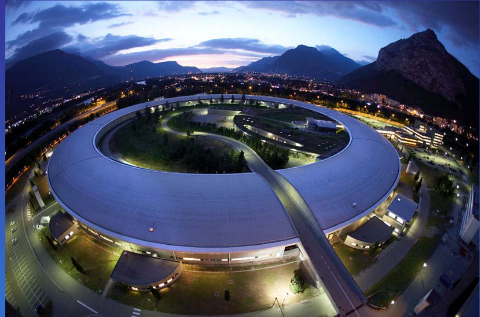
ESRF high energy 3 rd generation source
