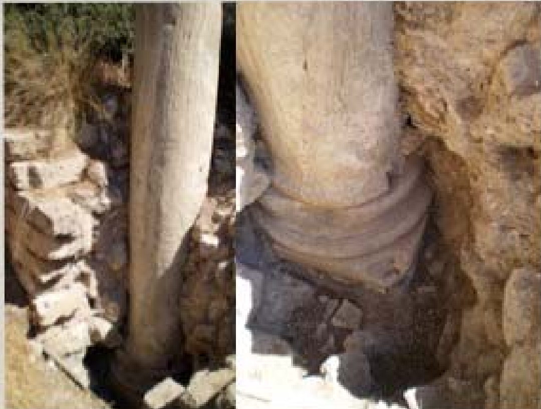
tilting ( \sim 10^\circ ), damaged pedestal
