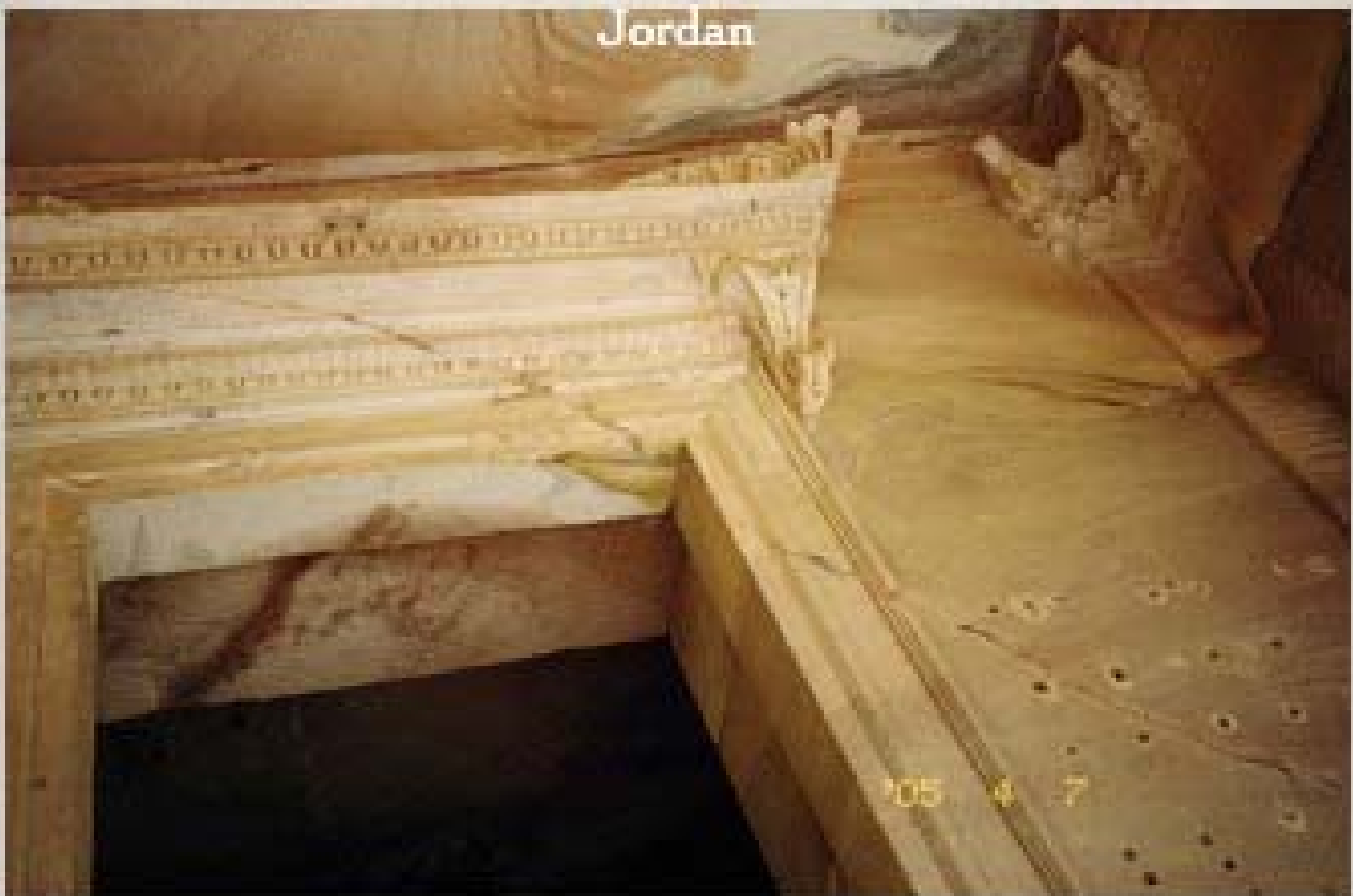
cracks through bedrock
