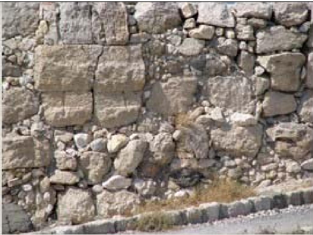
through-going cracks
