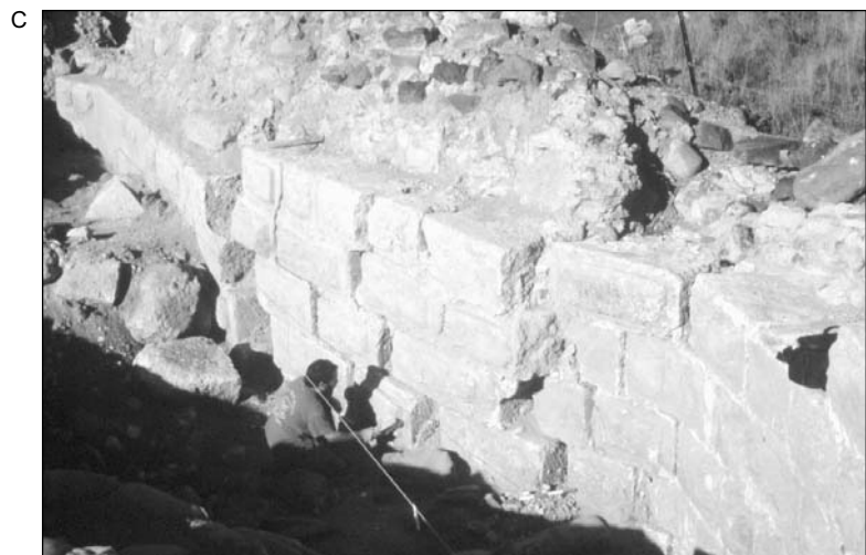
Figure 2. Location of offset human-made linear structures. A. Plan of Vadum Jacob fortress. Solid lines mark well-exposed parts of walls; dotted lines denote unexposed or partly exposed walls. B. Map of southern wall showing displacements and rotations of masonry. C. Photo of deformation in northern wall of Castle of Vadum Jacob. Line marks pre-faulting location of wall.
