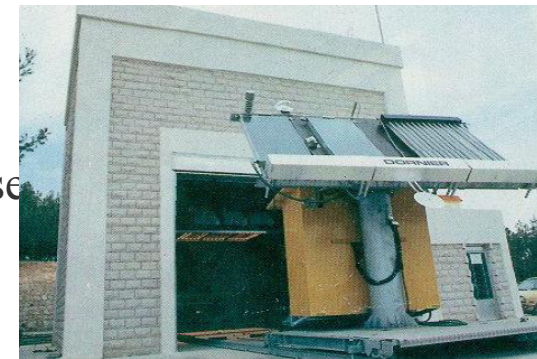
Solar Collectors indoor-outdoor testing facility
