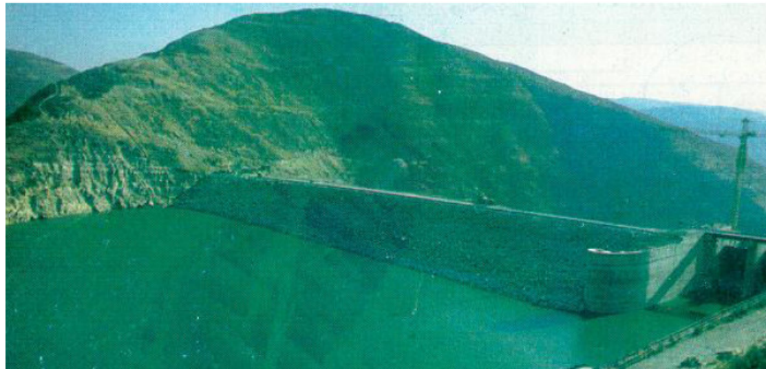
The King Talal Hydro Power Station
