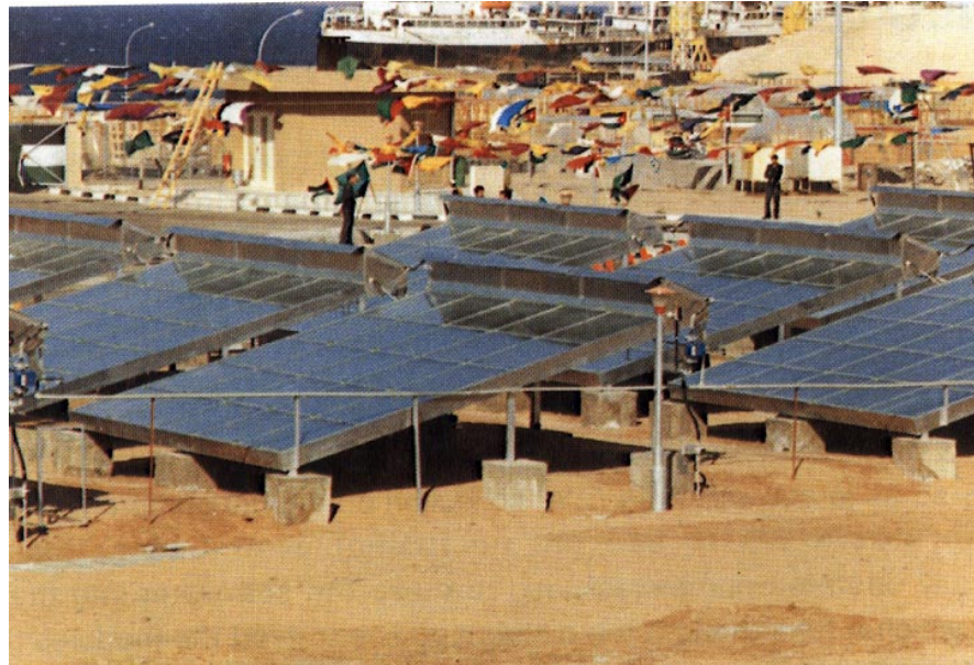
Solar desalination using solar heat pipe principle
