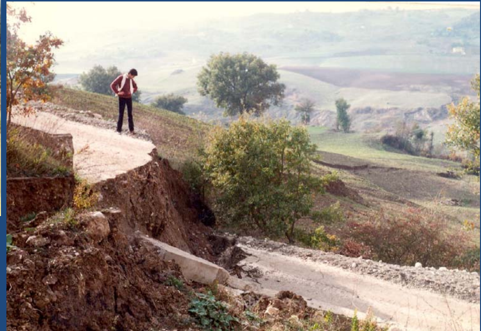
November 23, 1980 Irpinia-Basilicata, Italy earthquake ( M_s = 6.9 ). S. Giorgio La Molara: coseismic reactivation of a landslide
