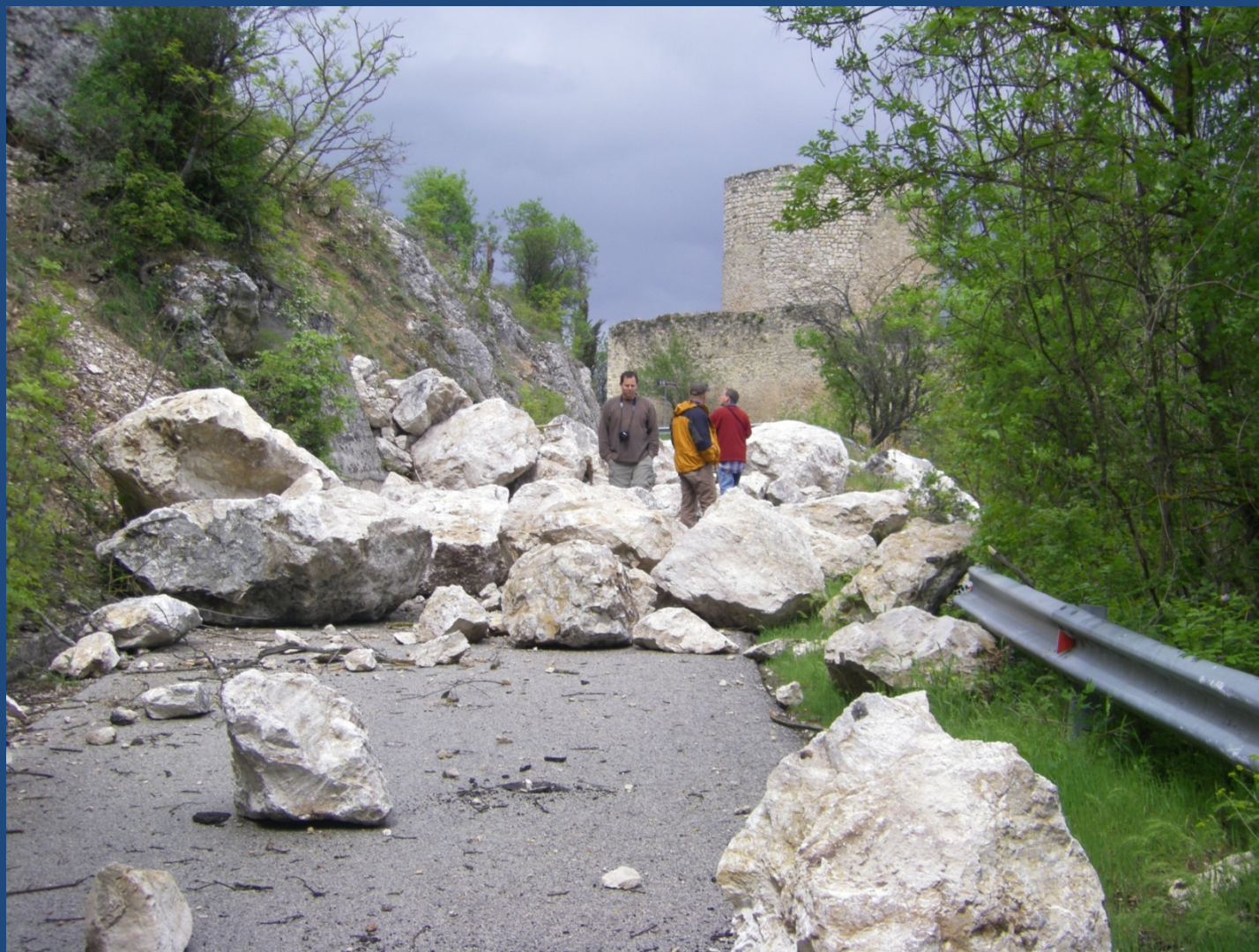
2009 April 6 th L'Aquila earthquake
