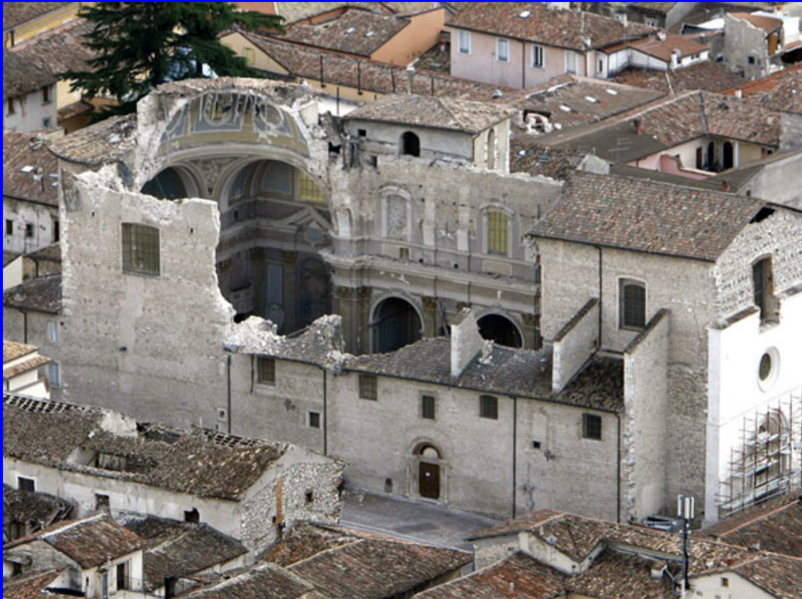
ABRUZZO EARTHQUAKE OF APRIL 6, 2009 L'Aquila, Santa Maria Paganica Church
