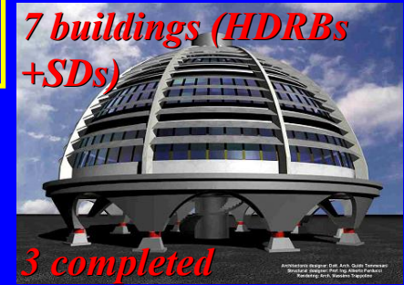
Civil Defense Center, Foligno: main building under construction (10 HDRBs, safety certification of A. Martelli)
