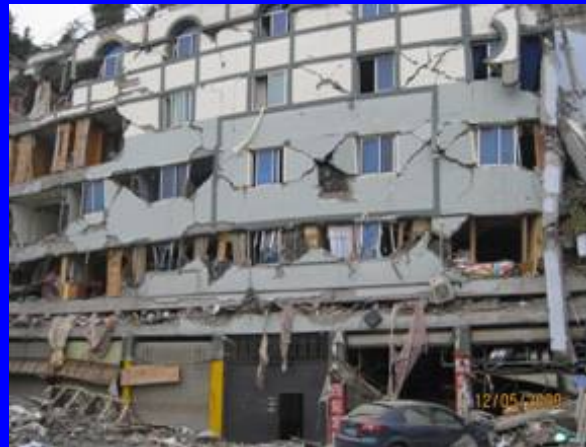
Collapse and heavy damage of conventionally founded buildings
