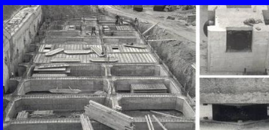
Telecom Italia Regional Center of Marche Region, 1 st Italian large building application of SI (5 buildings, 8 storeys, h = 25 \text{ m} , 297 HDRBs, 1991)
