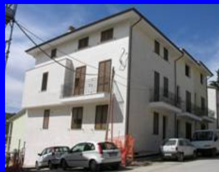
New private house, San Giuliano di Puglia (13 HDRBs + 2 SDs, 2007)
