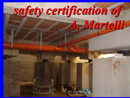
House at Fabriano, damaged by the 1997 earthquake (56 HDRBs, 2006)
