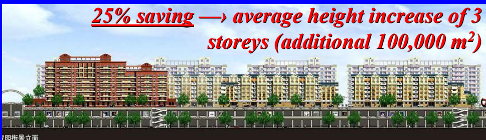
New Beijing residential centre : 50 isolated buildings (7-9 storeys, 480,000 m 2 ) on an unique 2-storey sub-structure (1500 m · 2000 m), with all infrastructures
