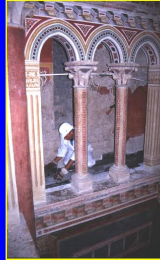
Installation of the 47 SMADs (1999) Installation of the 34 STUs (1999)
