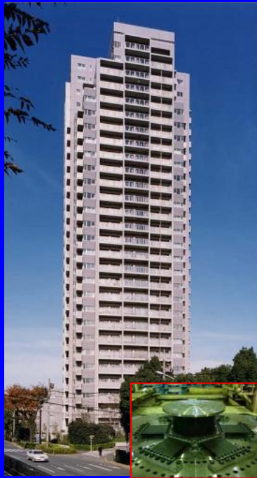
87.4 m building, Tokyo (2000): 30 LDRBs + 99 EPDs, T=4 s; anti-uplift
