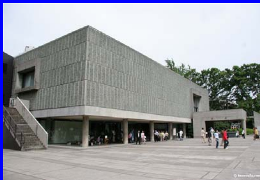
Retrofits began at the end of the years 1990s
