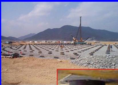
Inchon, South Korea, 3 tanks each with 392 HDRBs
