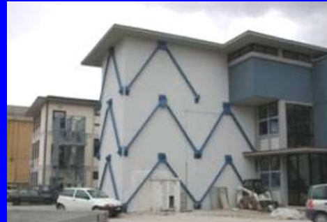
Retrofit with VEDs of the Gentile Fermi school (damaged by the 1997-98 Marche and Umbria earthquake) in Fabriano (Ancona), zone 2 (2000)
