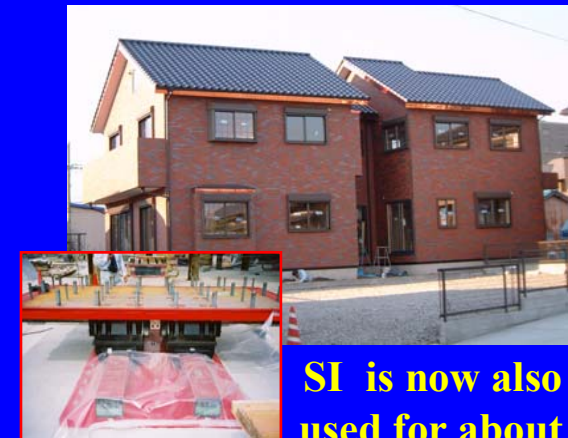
SI is now also used for about 3,000 private houses, even of small sizes (e.g. with sphere isolators, coupled with viscous dampers (VDs) and re-centering devices)
