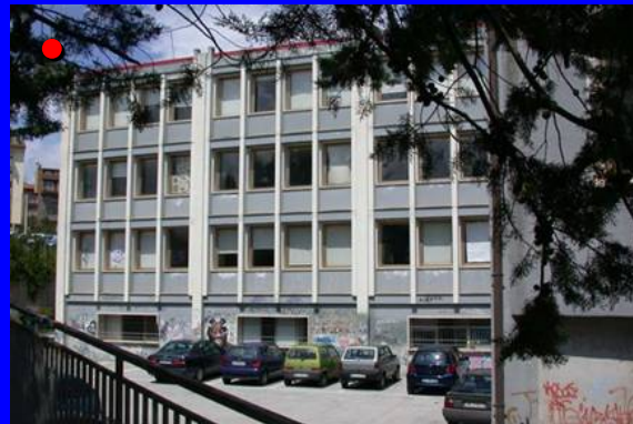
Romita High School, Campobasso (1300 students), zone 2 (demolition & reconstruction is beginning)
