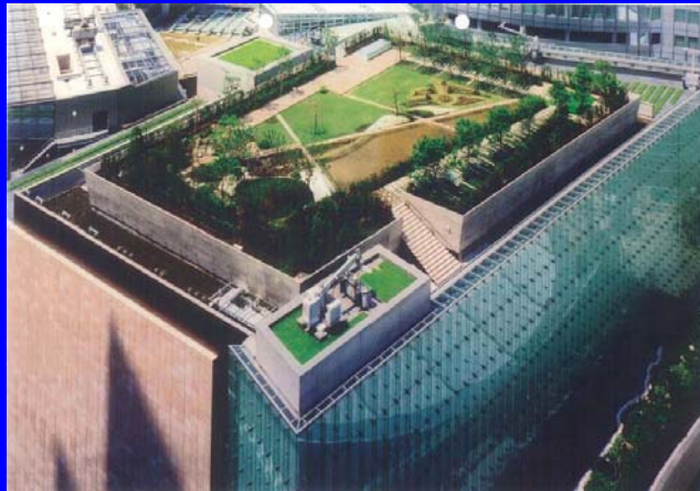
Roof garden (Green Mass Damper or GMD) used as “Tuned-Mass Damper” (TMD)
