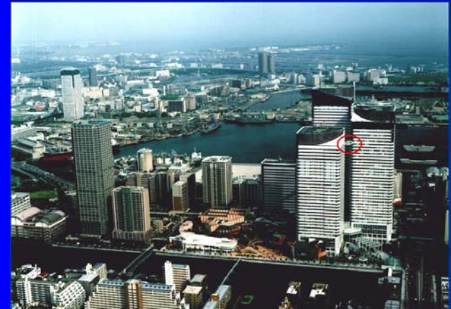
Active dissipation bridge (ADB) between high rise buildings
