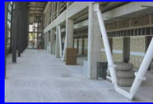
Costruction of the new Polytechnic University of Marche (r.c. prefabricated structure), Ancona, zone 2 (86 BRBs, 2006)
