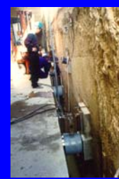
Telecom Italia Regional Center of Marche Region, 1 st Italian large building application of SI (5 buildings, 8 storeys, h = 25 \text{ m} , 297 HDRBs, 1991)
