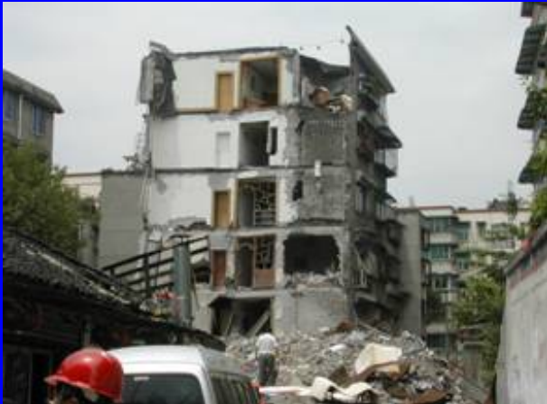
Collapse and heavy damage of conventionally founded buildings
