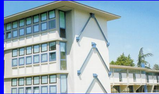
Retrofit with VEDs of the Gentile Fermi school (damaged by the 1997-98 Marche and Umbria earthquake) in Fabriano (Ancona), zone 2 (2000)
