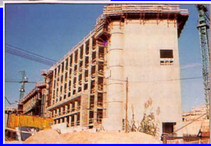
Telecom Italia Regional Center of Marche Region, 1 st Italian large building application of SI (5 buildings, 8 storeys, h = 25 \text{ m} , 297 HDRBs, 1991)
