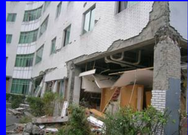
Collapse and heavy damage of conventionally founded buildings
