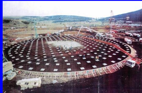
Revithoussa, Greece, years 1990s, 2 tanks ( \Phi = 20\text{ m} , at 70 m under ground level) each with 212 FPSs
