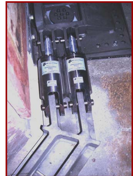
Viscous Dampers (VDs) "Shock Transmitter Units" (STUs)
