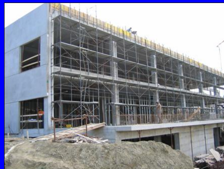
Costruction of the new Polytechnic University of Marche (r.c. prefabricated structure), Ancona, zone 2 (86 BRBs, 2006)
