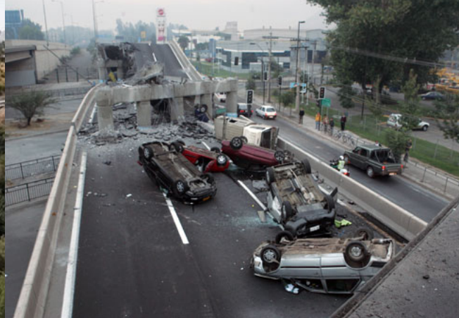
Reinforced concrete bridge
