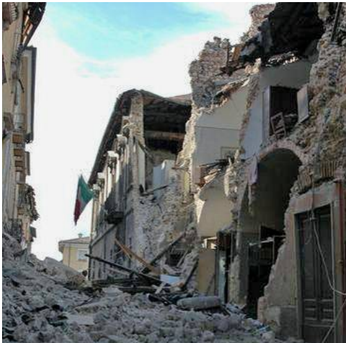
Masonry collapse
