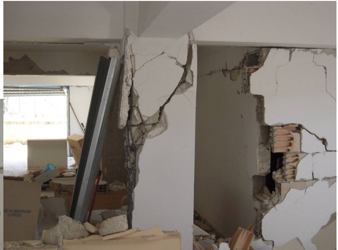
Shear failure
