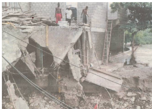
Reinforced concrete floor
