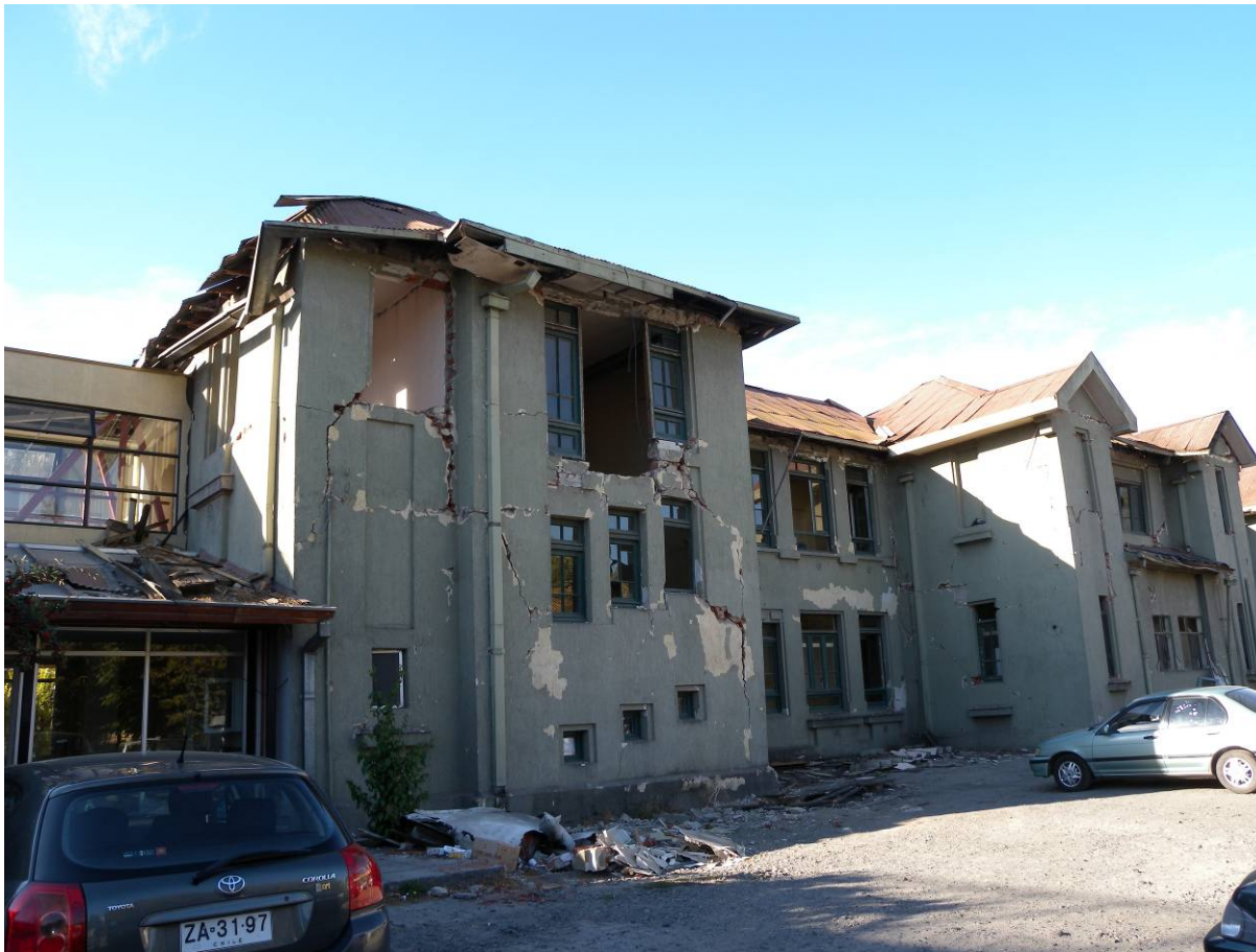
Talca, Hospital Viejo, to be demolished
