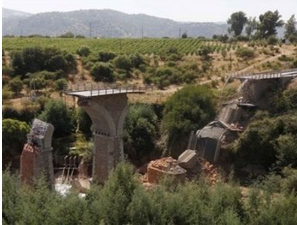
Historic masonry bridge
