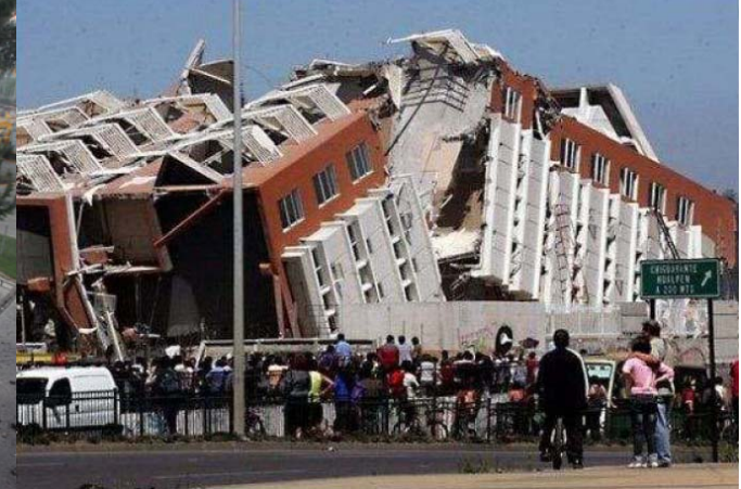
RC Building collapse
