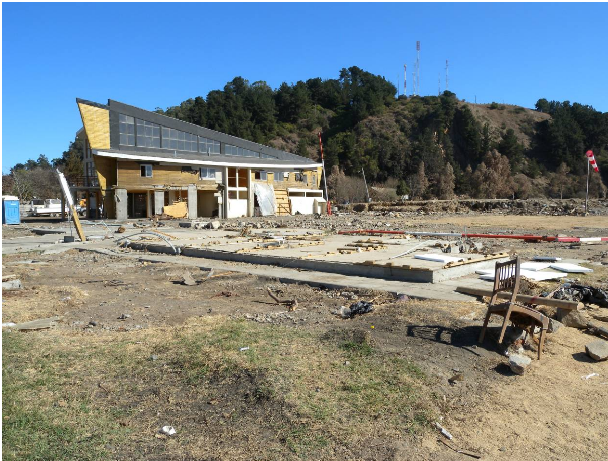
Constitucion. Reinforced concrete building survived the tsunami
