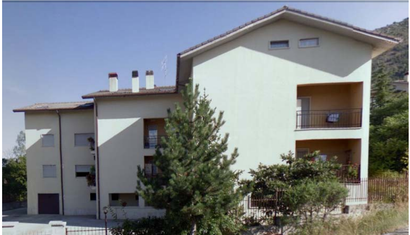
Building in via Dante Alighieri 2 Before earthquake
