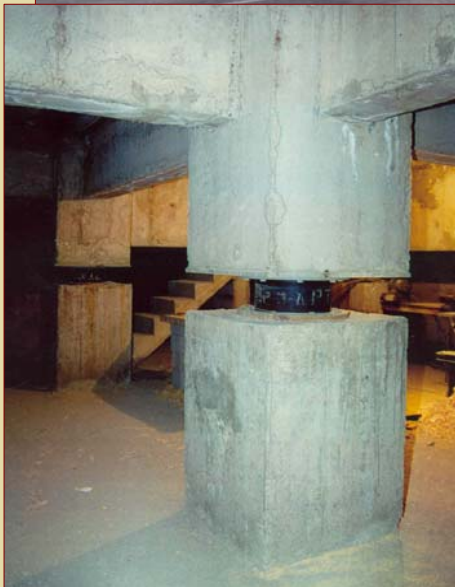
Newly constructed 4-story base isolated apartment buildings in Gyumri.
