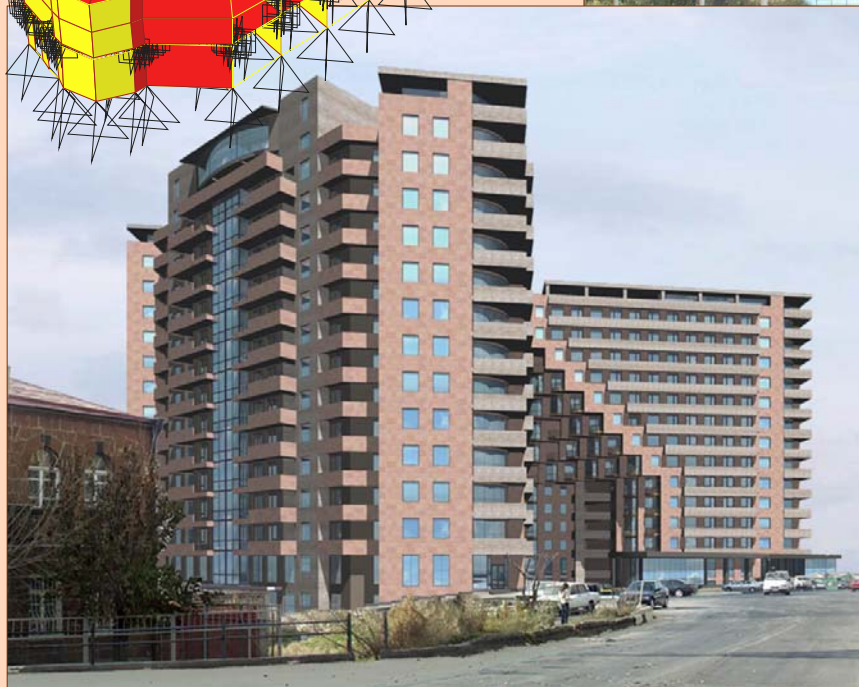
Newly constructed 15-story base isolated buildings of the multifunctional residential complex “Northern Ray” in Yerevan
