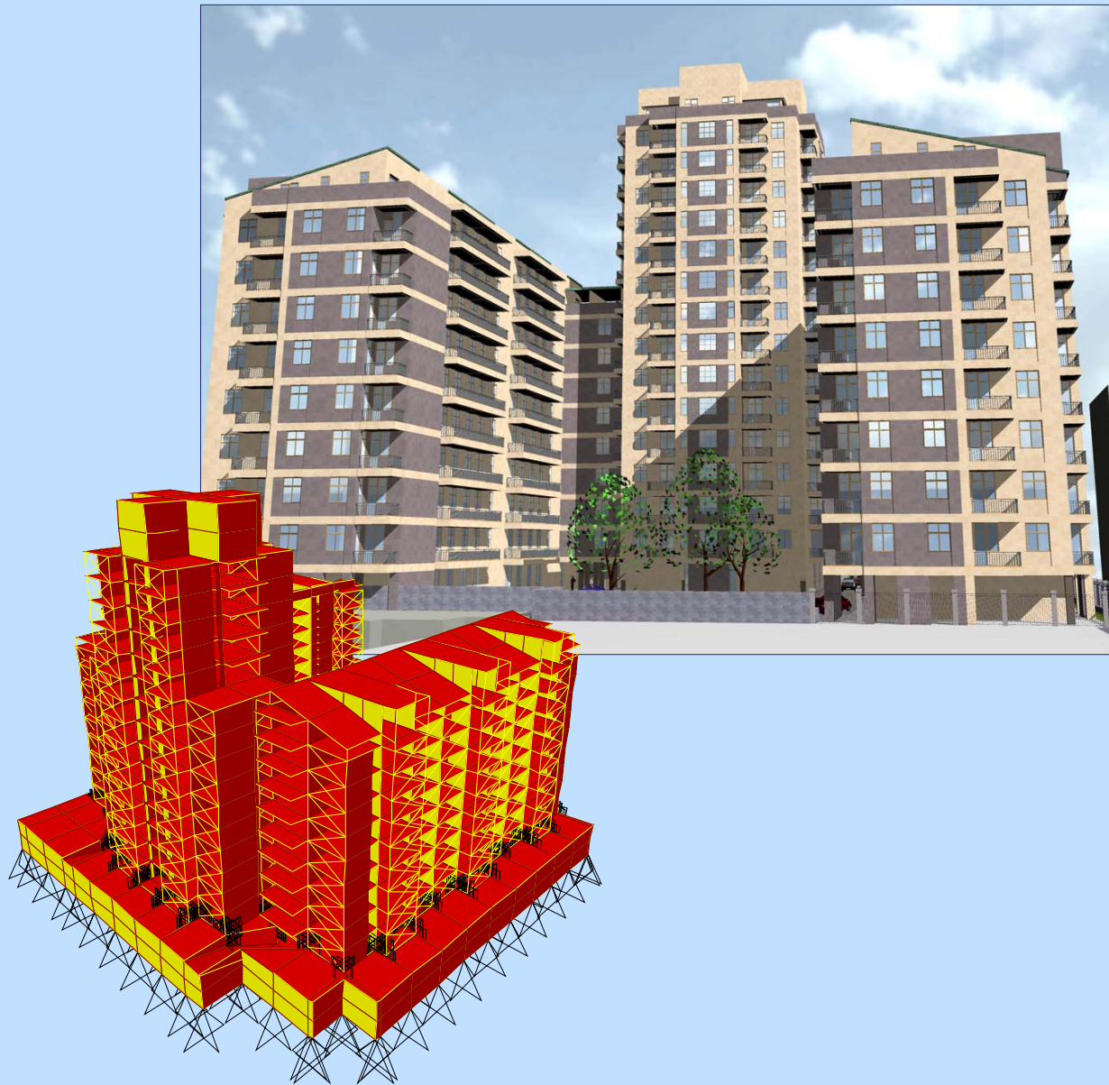
Newly constructed 16- and 10-story base isolated buildings of the multifunctional residential complex “Our Yard” in Yerevan
