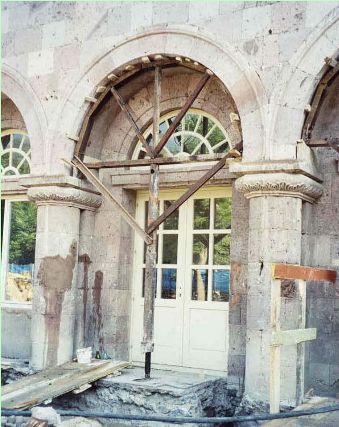
Temporary support under the existing arches
