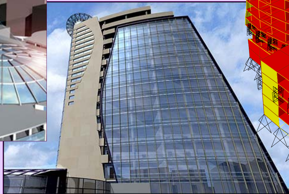
Newly constructed 20-story base isolated “Elite Plaza” business center building in Yerevan
