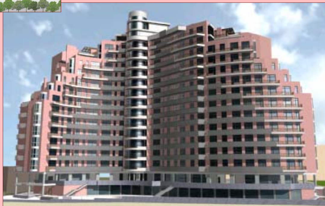
Newly constructed 15- and 13-story base isolated buildings of the multifunctional residential complex “Dzorap” in Yerevan
