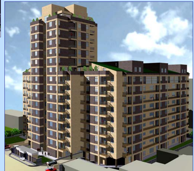
Newly constructed 16- and 10-story base isolated buildings of the multifunctional residential complex “Our Yard” in Yerevan
