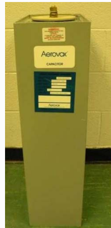
Capacitor 20 kv, 200KA
