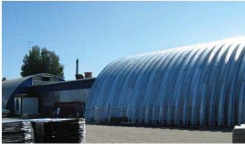
real object - part of a warehouse complex, 12m span and 45m length
