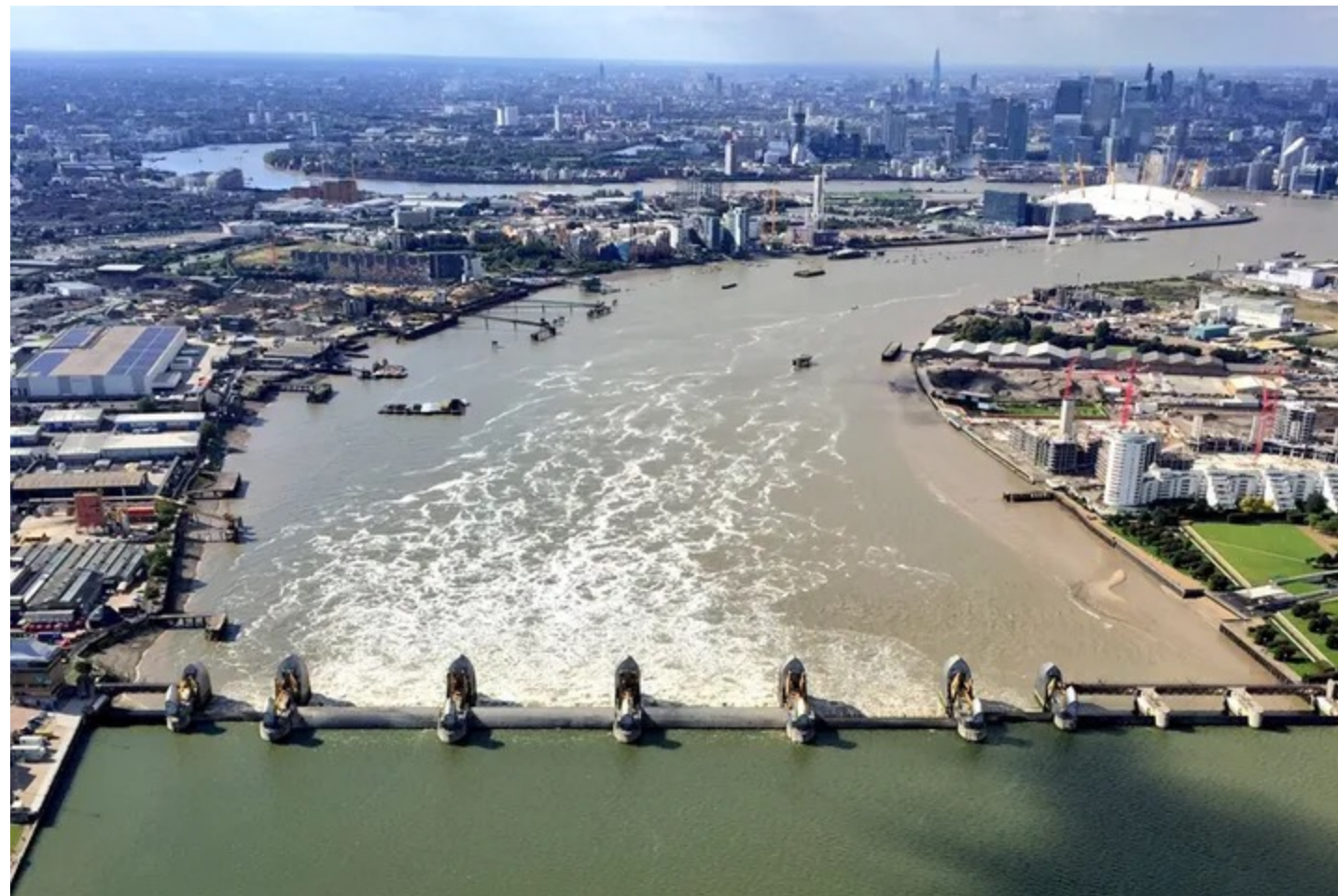
Aerial view of the Thames Barrier with closed gates (National police air service/ gov.UK)
