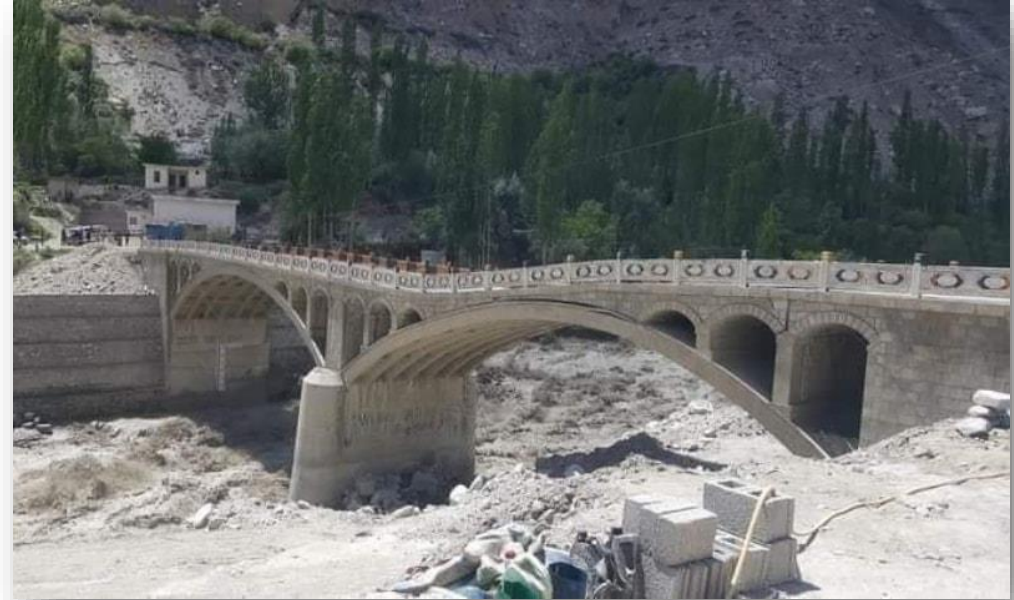
Damaged bridge at Hassanabad, after May 2022 GLOF
