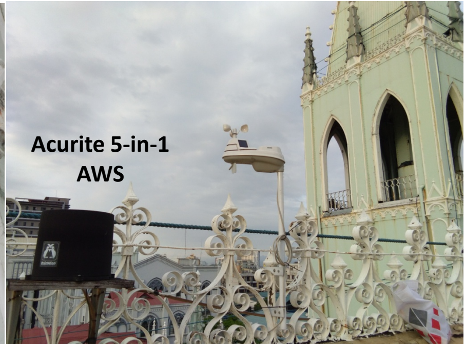
THVDR6 – Basilica's Roof
