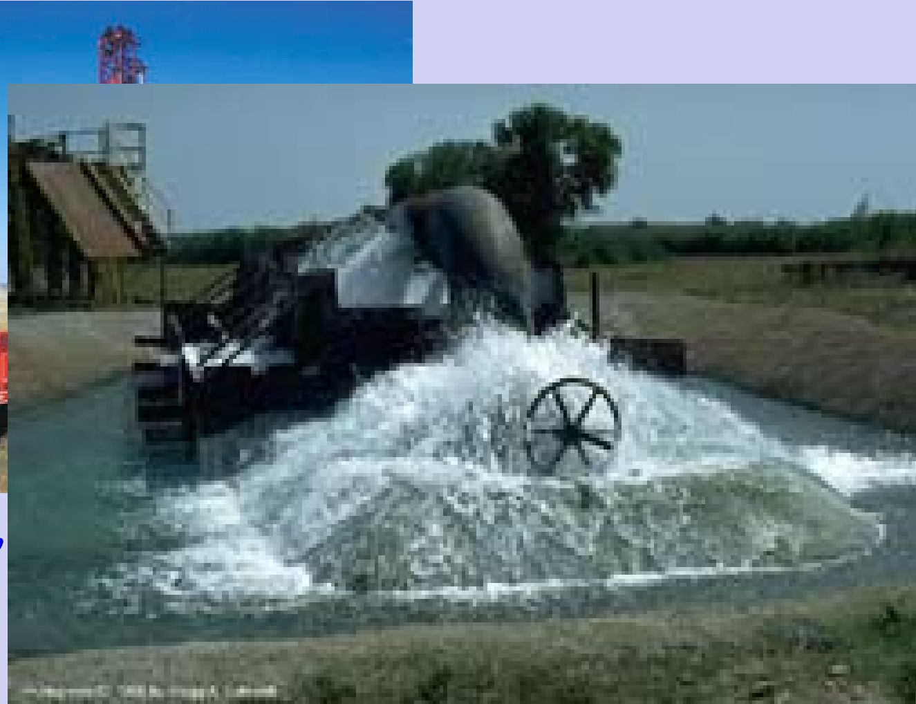
Mechanical Pumps: Ground Water Over Pumping
