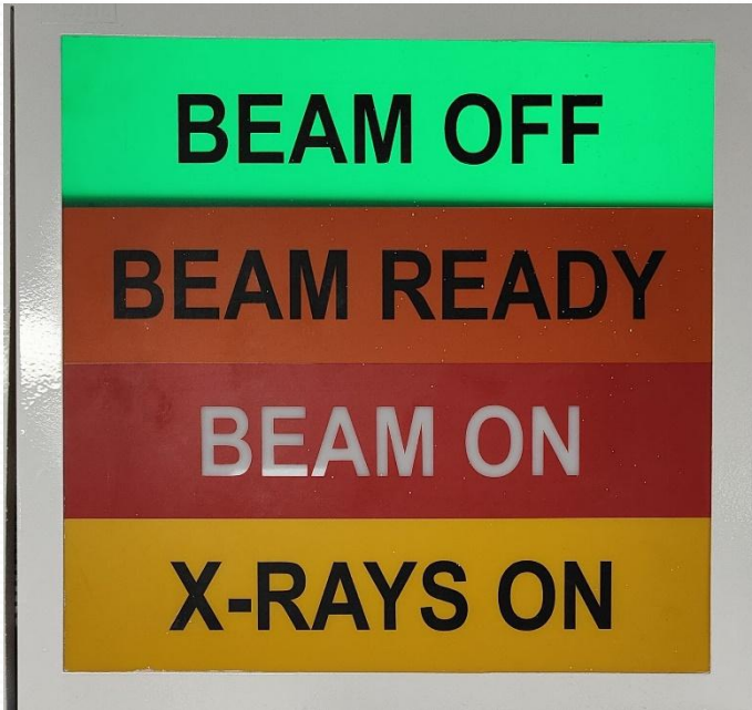
X-Ray ON Indicator Near treatment Door
