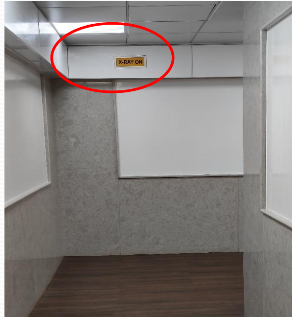
X-Ray ON Indicator in Maze Wall
