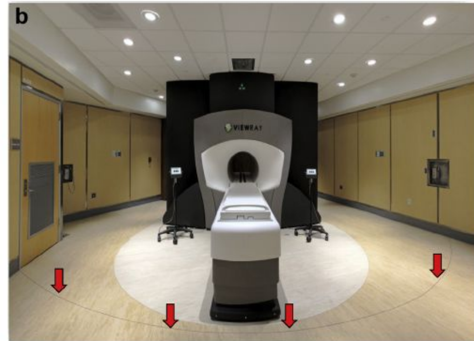
Figure 1 (a) Fringe field strength of 0.35T and 1.5T magnetic resonance imaging along the B_0 direction as a function of the distance from isocenter. (b) Picture of a magnetic resonance-guided radiation therapy vault with the 5 Gauss line clearly marked on the floor as being a potential hazard.
