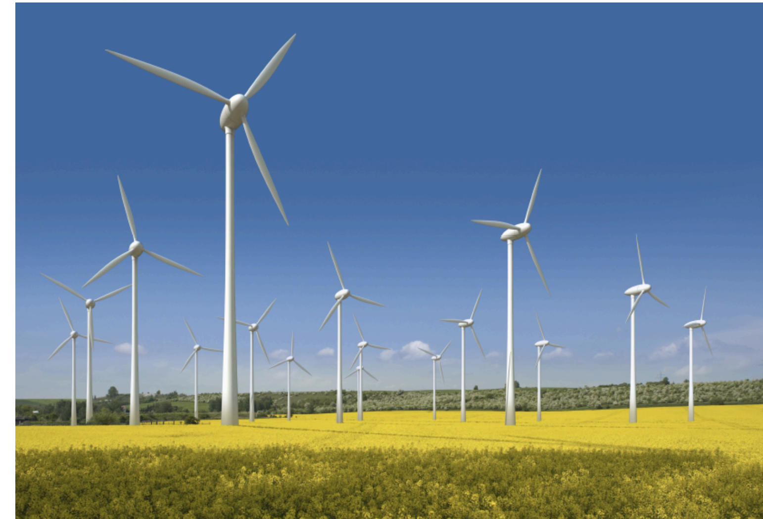
Magnets for generators
