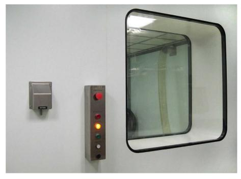
In order to maintain air quality, windows in controlled contamination environments must not be openable. To guarantee the view towards the outside or between rooms, windows made of a double layer of glass are used, fixed on an aluminum frame and sealed
