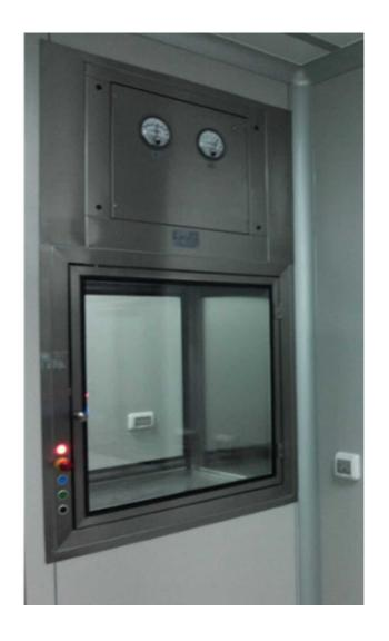
Differential pressure gauges and other display for visualizing the parameters of the clean room are typically wall mounted and allow for continuous monitoring of correct set point and operation of the ventilation system.
