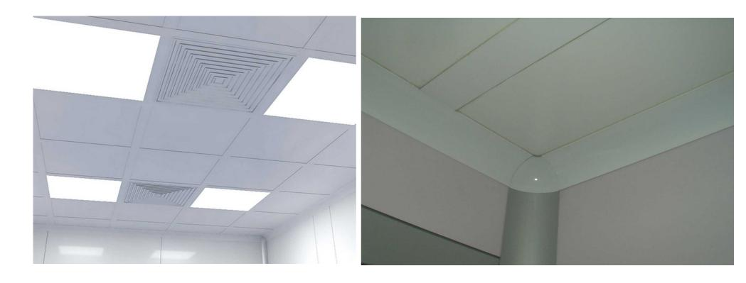
The pharmaceutical grade ceiling is made of plastic laminate or aluminum, welded and disinfectable.
