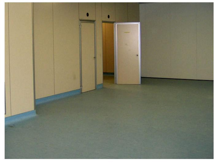
The floor must also be suitable for a controlled contamination environment. Homogeneous vinyl floors are usually made, with PVC finishes on the surface of the floor itself.
