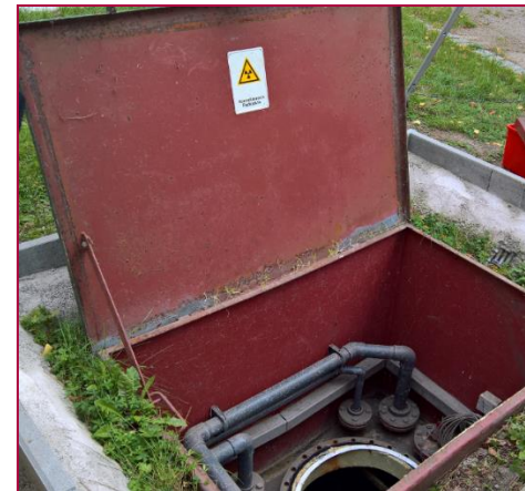
Plant for decay of radioactive waste water with underground tanks
