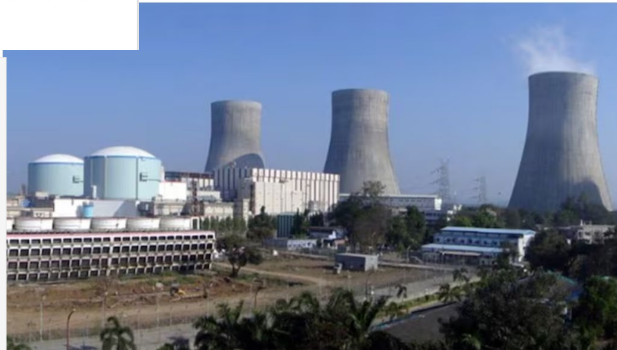
The 500 MWe Prototype Fast Breeder Reactor at Kalpakkam in Tamil Nadu, designed and built entirely in India by BHAVINI and IGCAR, attained criticality on 6 April 2026. It is India's most advanced nuclear reactor to date.
