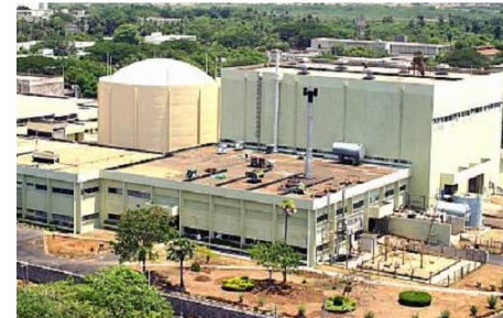
FBTR, 13 MW(e) India, 1985
