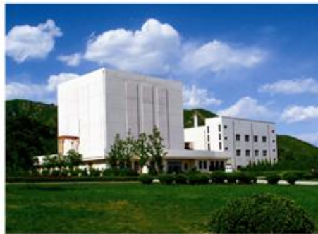
Test reactor (HTR-10, 1986)
