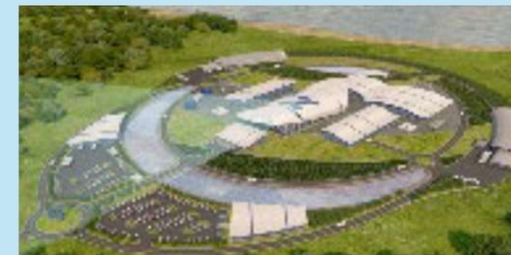
4. To the plant site
