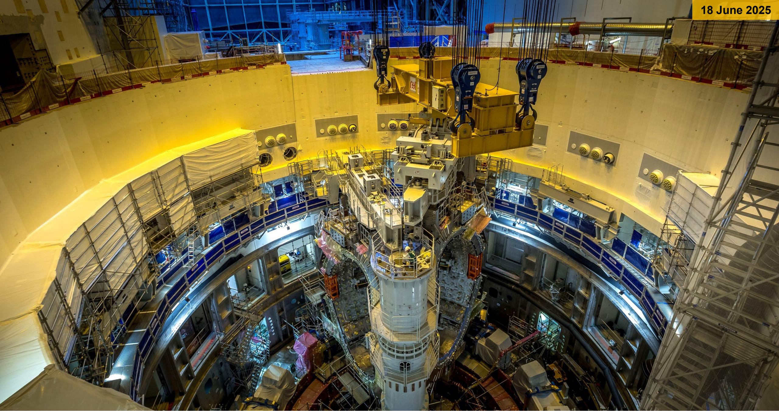
SM 6 being lowered into the pit
