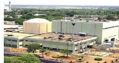
FBTR, 13 MW(e) India, 1985
