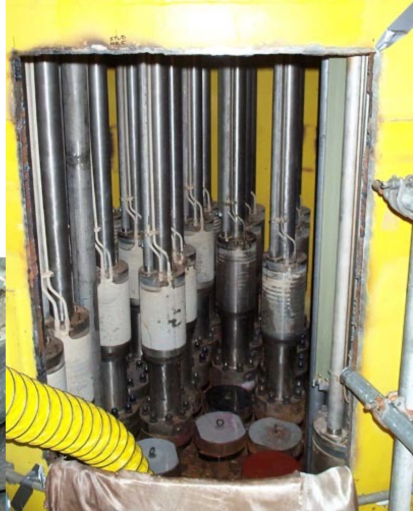
Control Rod Drive Mechanism in Place
