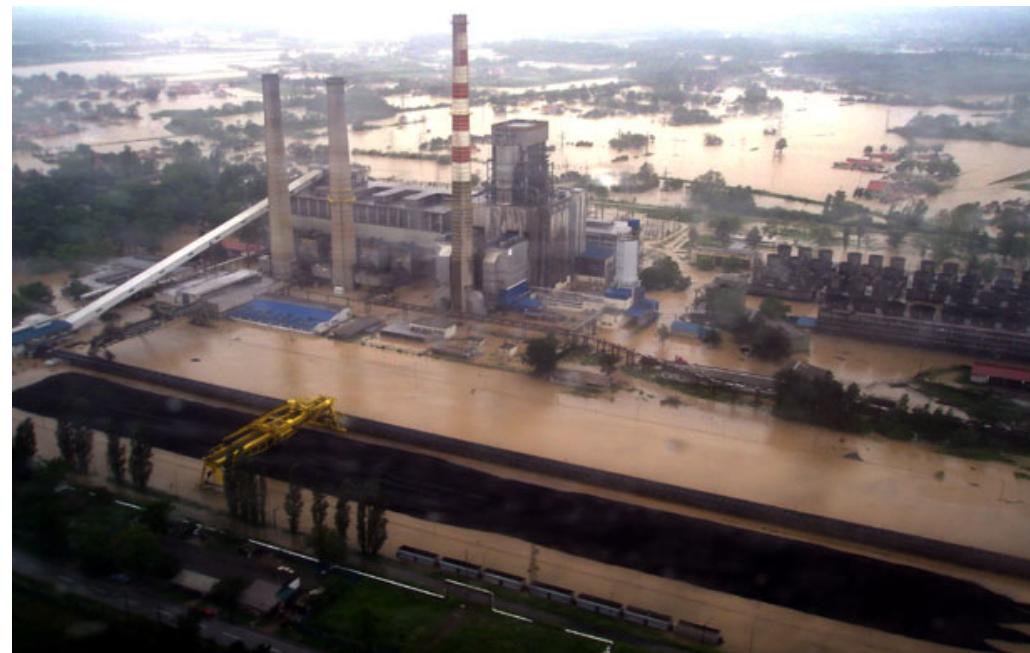
Figure 3. Thermo-power plant „Nikola Tesla“.
