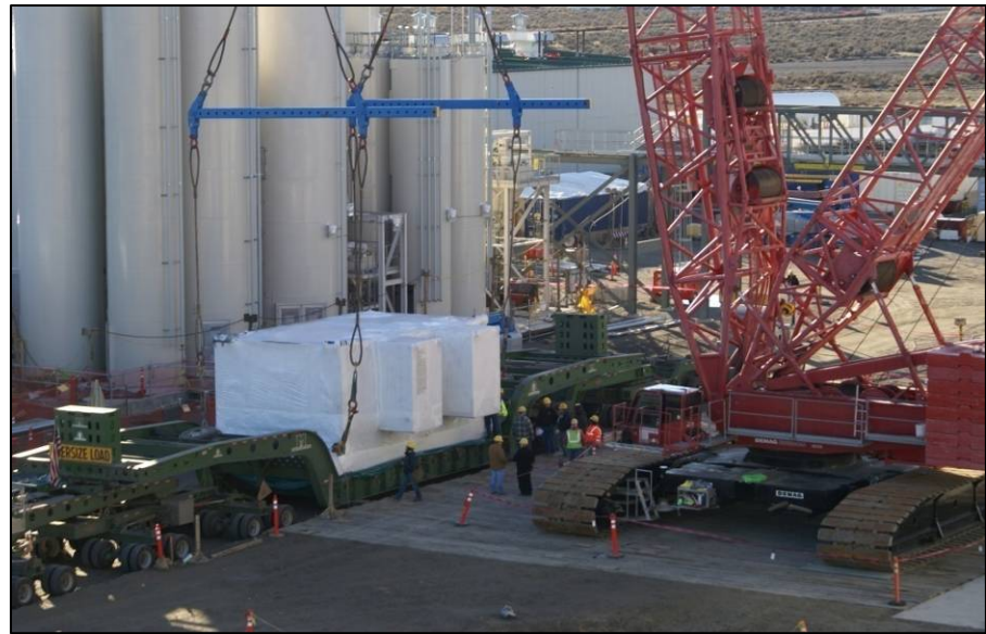
LAW Melter During Installation
