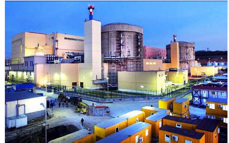
Cernavoda NPP in Romania: unit 1 & 2 (~700 MW) PHWR CANDU6 type
