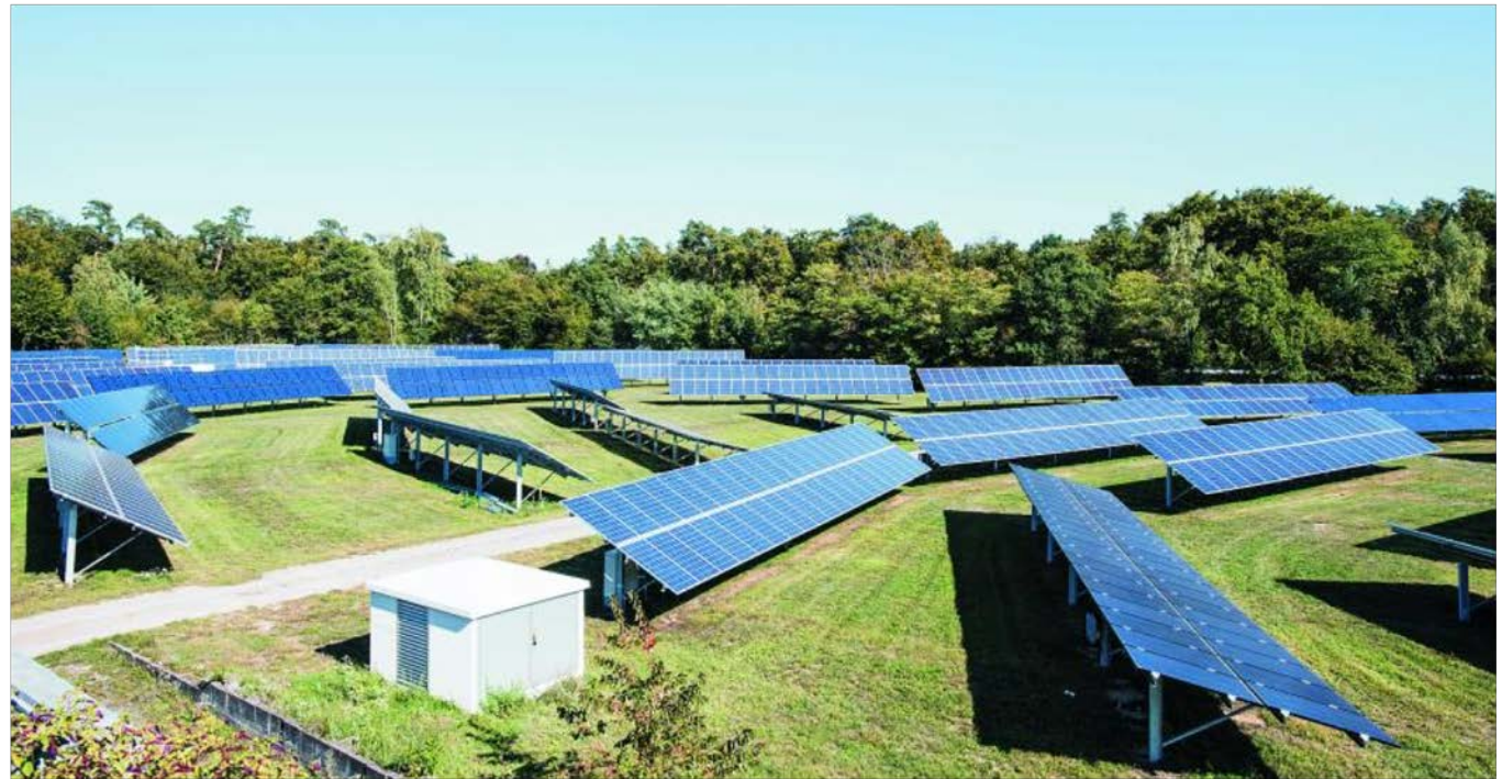
Measurements carried out at KIT will determine the effect of soiled solar panels on the output of photovoltaic systems caused by deposited mineral dust. (Photo: Sandra Göttisheim)
