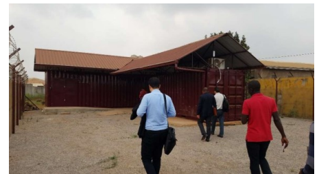
Fig. 2: External view of the Cameroon Interim Storage Facility
