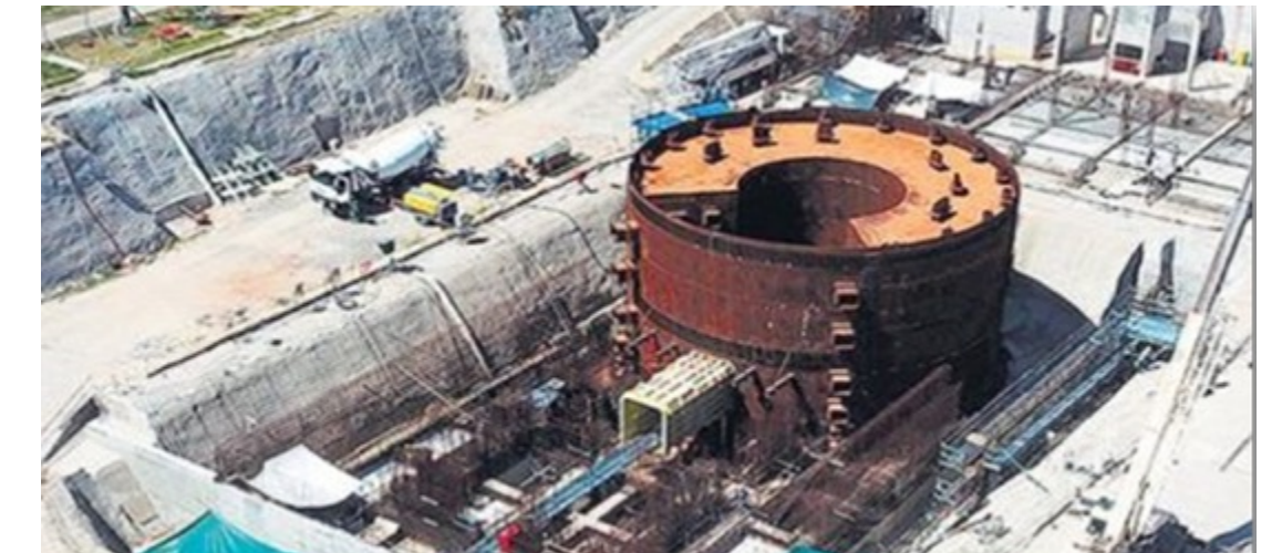
CAREM under construction, to start operation in 2023
