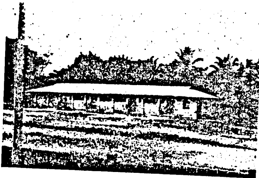
FIG. 12. MUDWALL WITH CEMENT PLASTER AND CORRUGATED IRON SHEET ROOFING.
