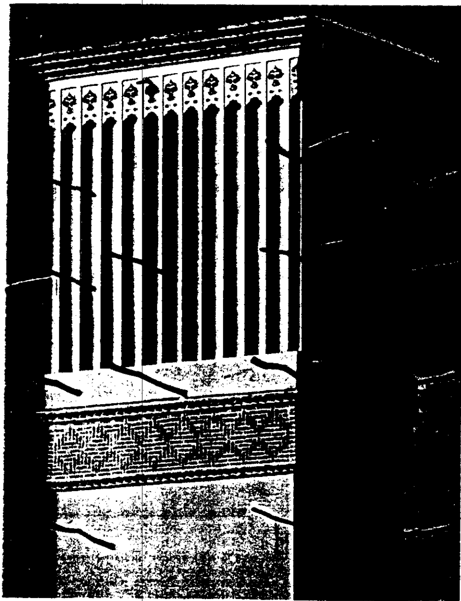
CLOSEUP VIEW OF THE TOP OF A WIND TOWER in Yazd shows the ends of its reinforcing beams. The tower is about 13 meters high and its openings are about three meters high. The tower in illustration on page 145 is about 34 meters high; its openings are about 11 meters high.
