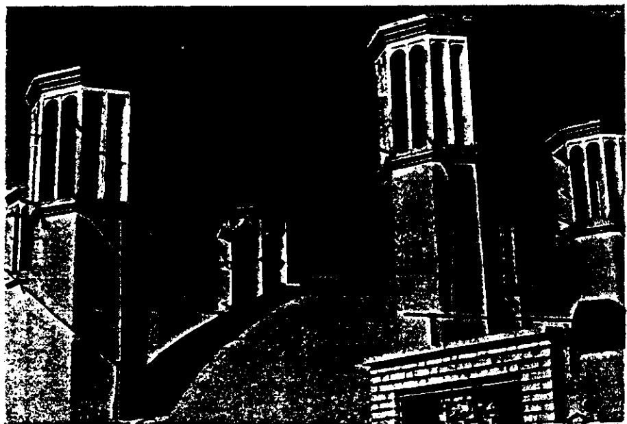
DOMED ROOF AND WIND TOWERS of a cistern in Yazd appear here. Towers are about 12 meters high; cistern is about 12 meters deep and can hold some 1,000 cubic meters of water.
