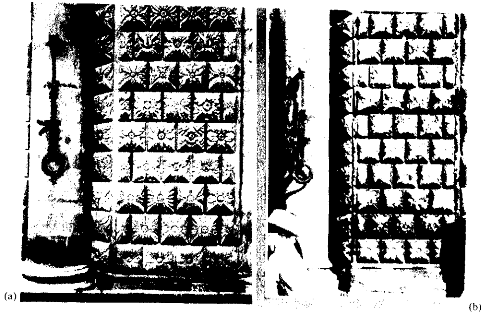
Fig. 1. Detail of the Palazzo Re Enzo, an example of a historical building in sandstone situated in the center of Bologna. On the left (a), the wall decoration as appeared in a photograph taken at the beginning of this century (from the Poppi archives, by kind permission of the Cassa di Risparmio di Bologna), on the right (b), the same detail as it appears as of 1988, where evident signs of damage can be seen.
