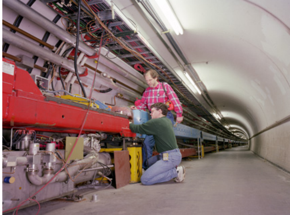
Tevatron tunnel with old Main Ring in place
