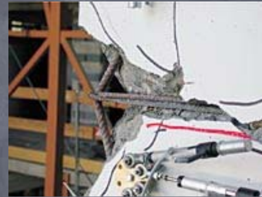
Identification of insufficient seismic detailing. tall pier A40, buckling of longitudinal reinforcement at h = 3.5\text{m}
