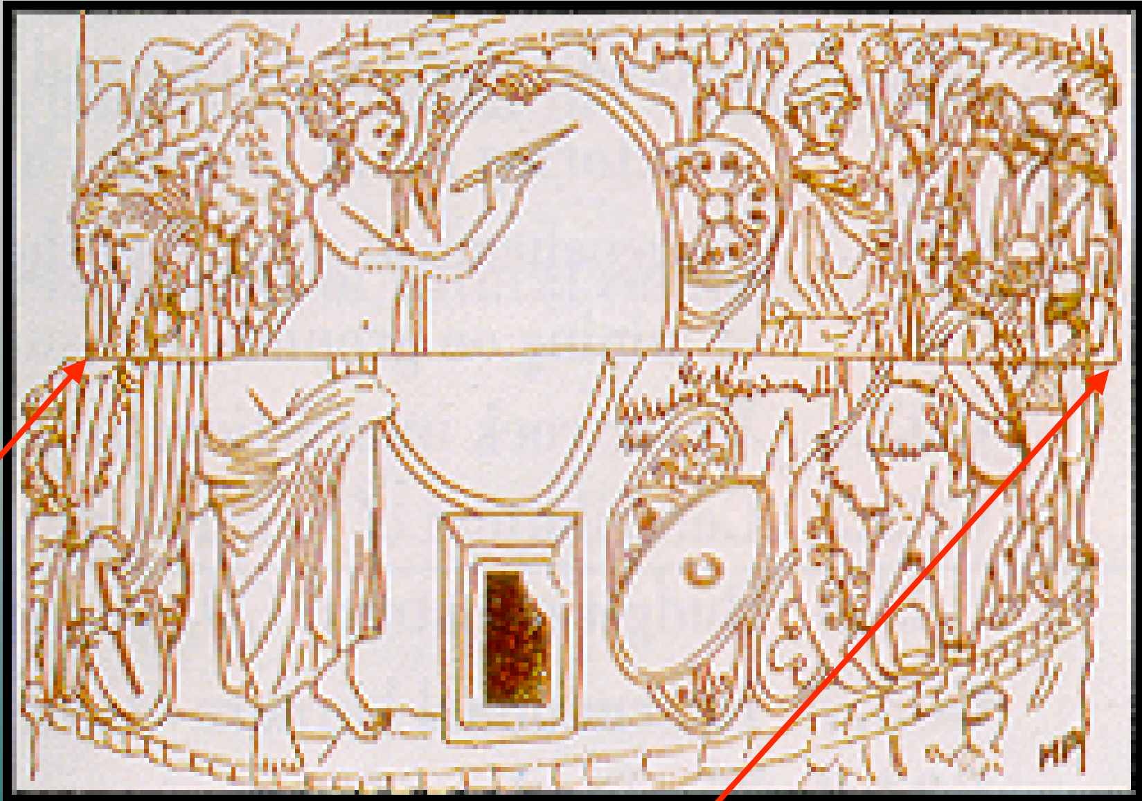
Dislocation of about 8 cm between rocchi IX and X of Colonna di Marco Aurelio (from ITALIA 2004, 32 nd International Geological Congress; 1 st Circular)
