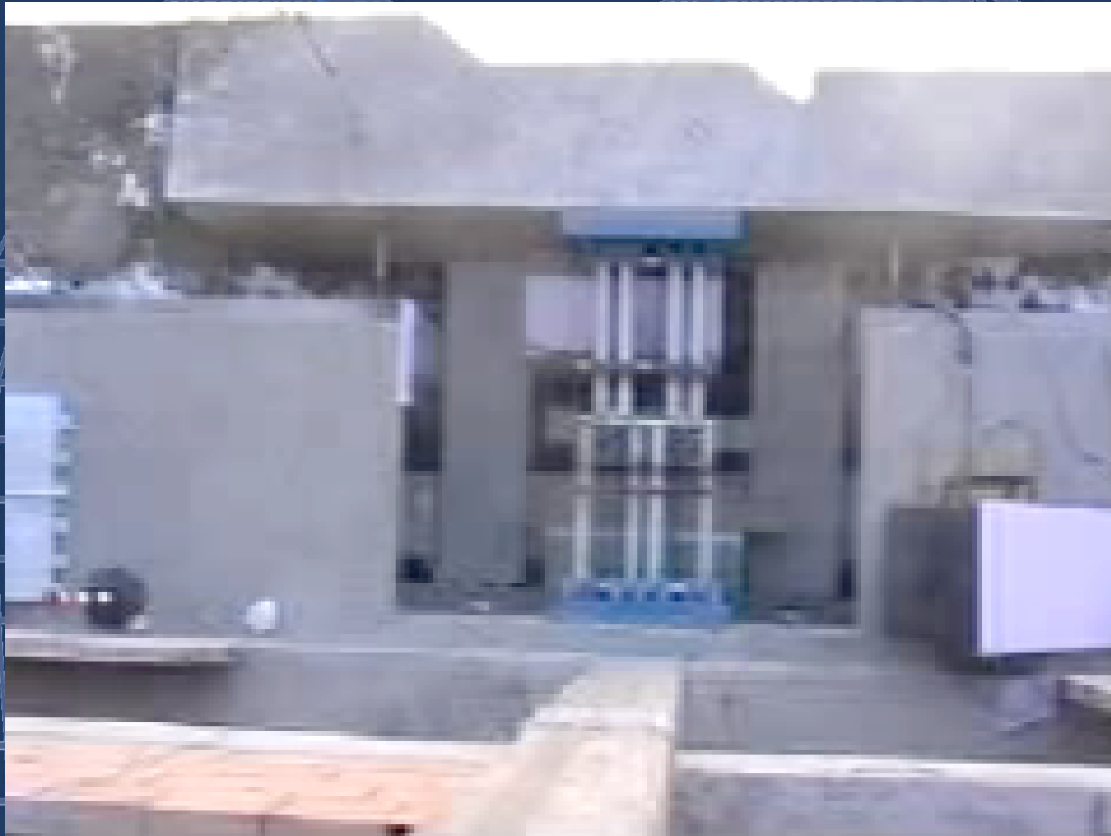
Dynamic test of a base isolated building in Rapolla ( Braga and Laterza, 2000 )
