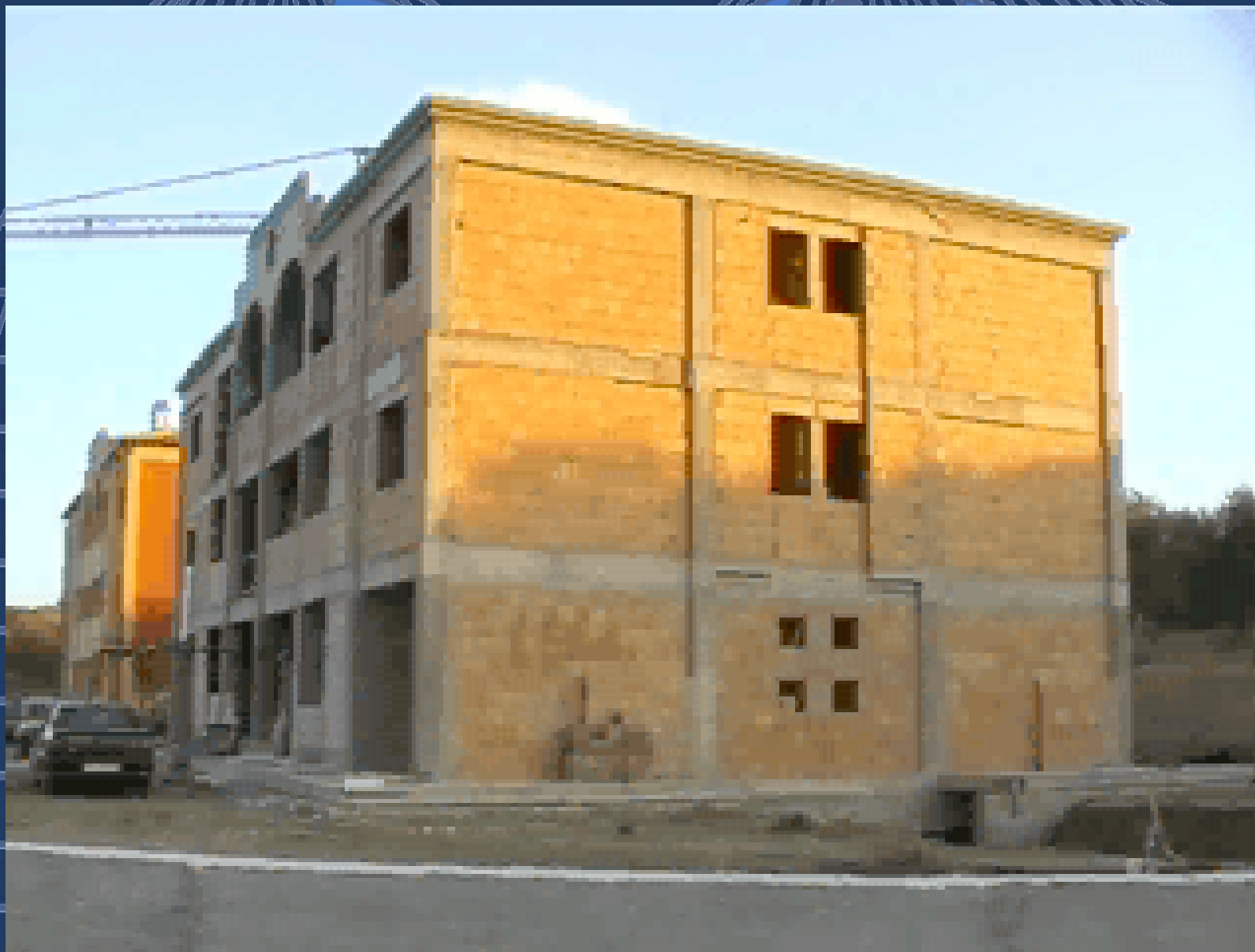
Dynamic test of a base isolated building in Rapolla ( Braga and Laterza, 2000 )
