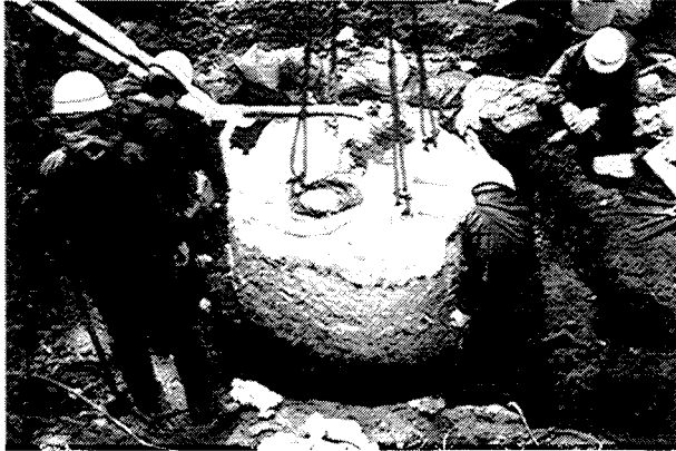
Freezing sampling performed at GL – 5m after excavation
