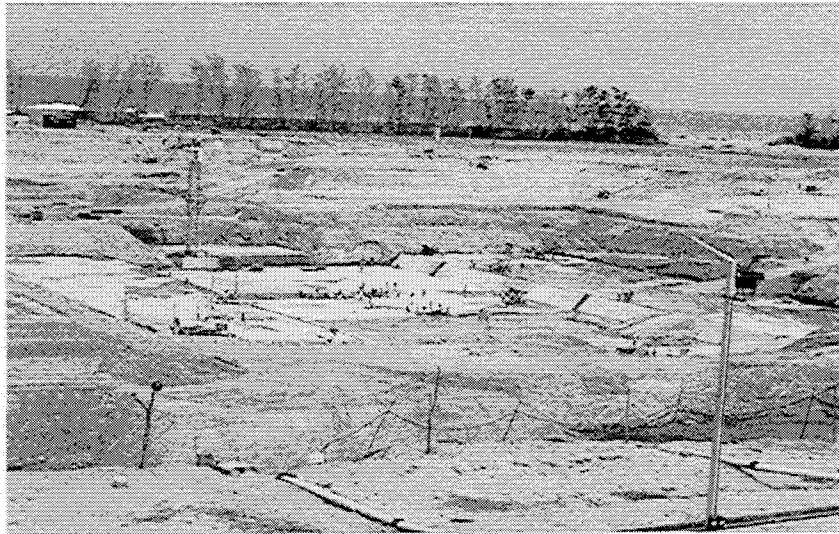
Excavated pit of FBR after mud mat
