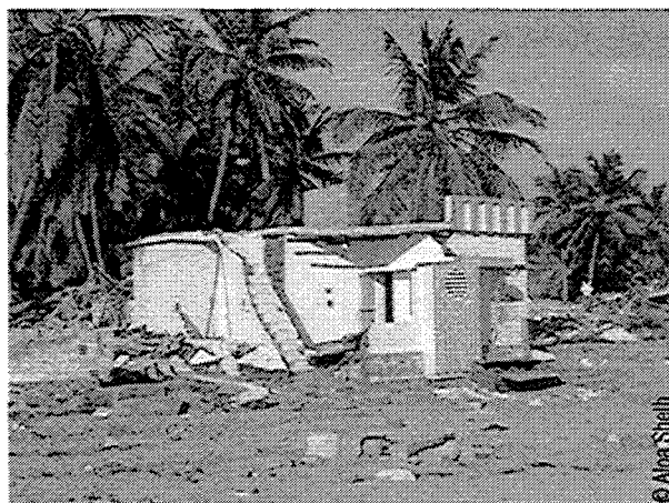
Partially damaged house
