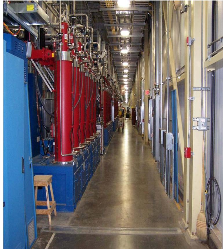
Warm linac: 7 – 2.5MW, 4 – 5MW klystrons
