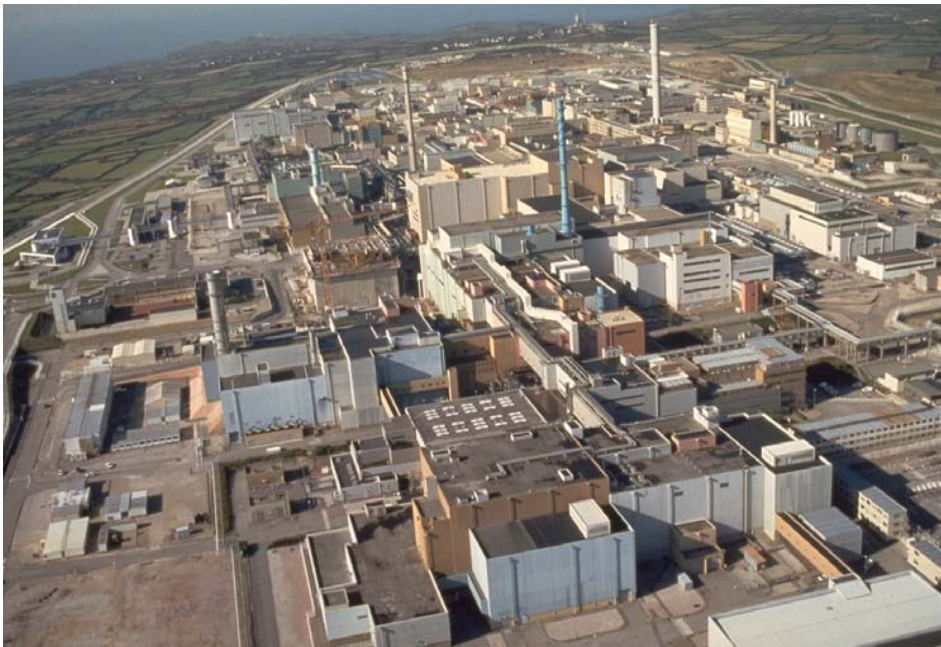
La Hague SF reprocessing facilities
