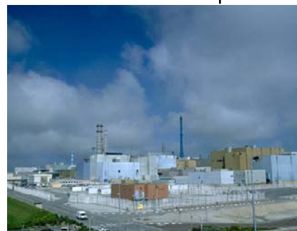
La Hague Plant
