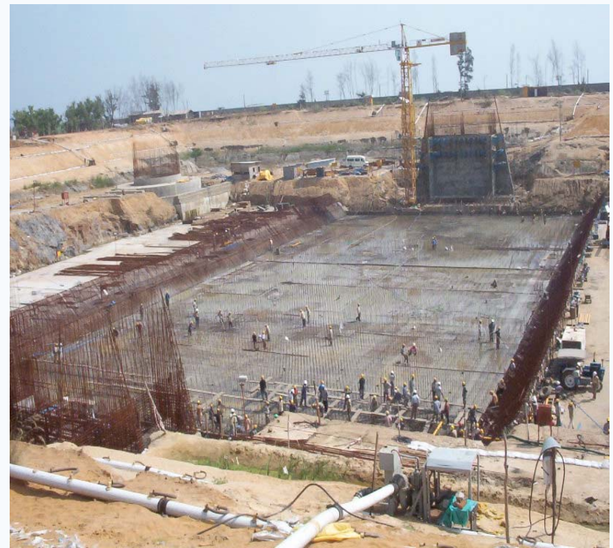
Construction site - India's 500 MWe Prototype FBR
