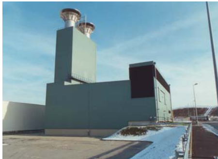
E/EV/SE storage facility at La Hague
