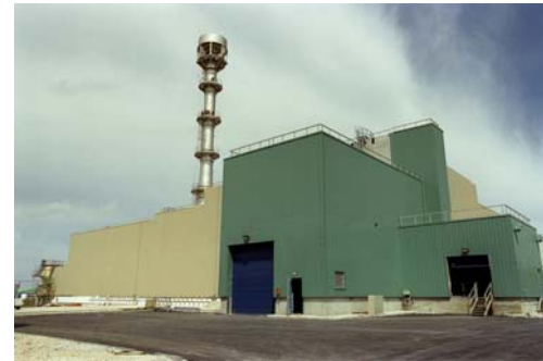
ECC storage facility at Marcoule
